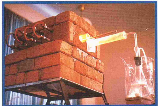
From the pioneer-period showing a home made diffusion furnace.
